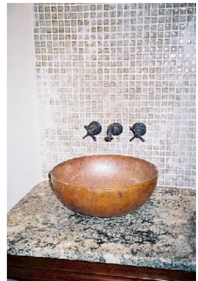
Guest powder room copper sink copper cistern with granite
