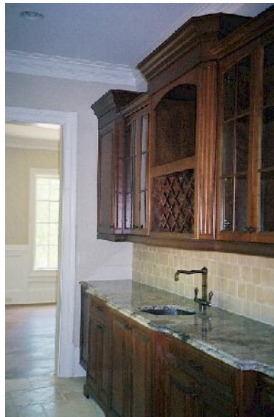
Butler pantry, sink, copper fixture granite counter top
